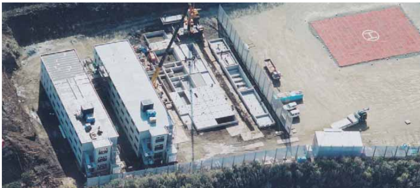
Izu Shelter under Construction
